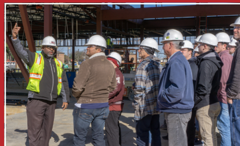
Hill International Consultant Marcus Swayzer speaks with LIT drafting students about the Eagles' Nest for Student Success construction process.
